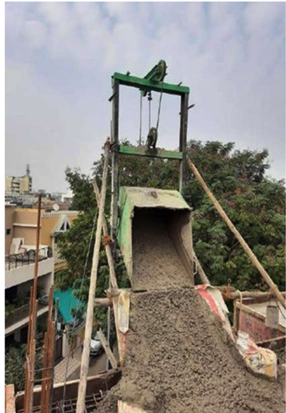
Fig. 4: Figure of real time elevator with hopper releasing concrete on floor
