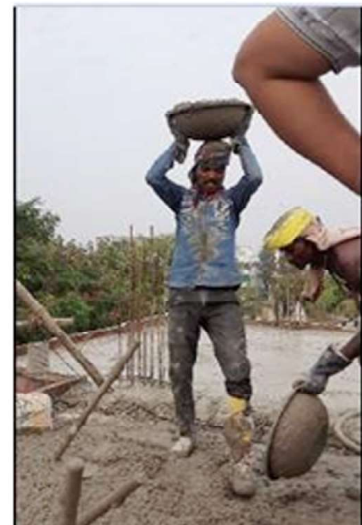
Fig. 6: (c): Lifting and holding Head-Pan on head POSTURE-3
