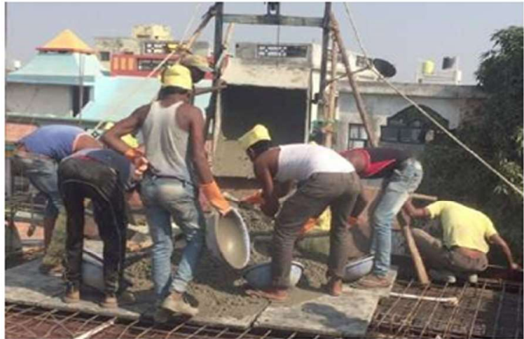
Fig. 5: Laborers collecting concrete in the iron-pan
