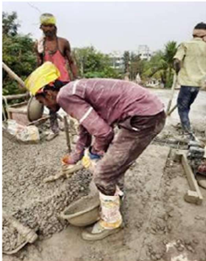
Fig. 6: (a): Collection of Concrete in the head-pan POSTURE-1
